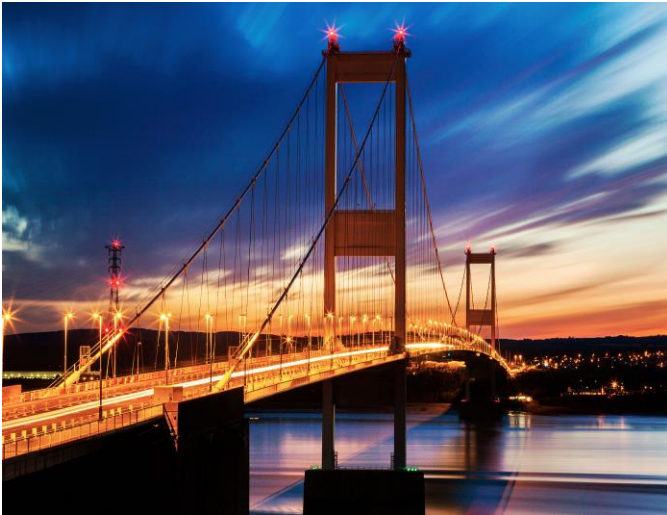
View of Severn Bridge
